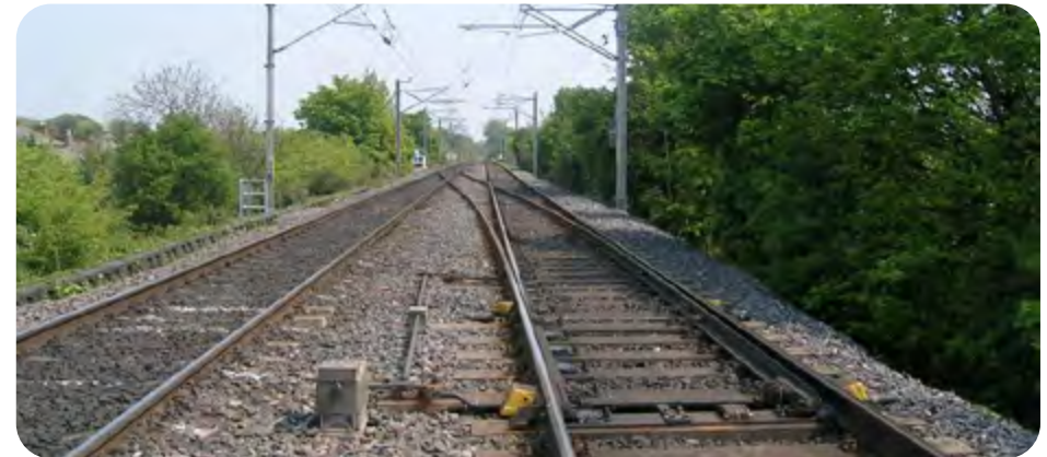
View of typical section of twin track electrified rail line
